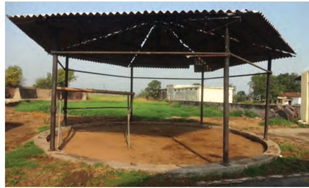
Fig. 1.18: Casting pit filled with sand as bedding material
