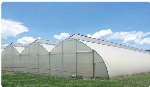
Fig. 7.4 Typical naturally ventilated polyhouse (NVPH)
