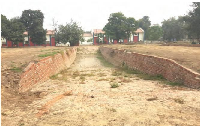
Fig. 1.9(a): Structure of bunker-type silo
