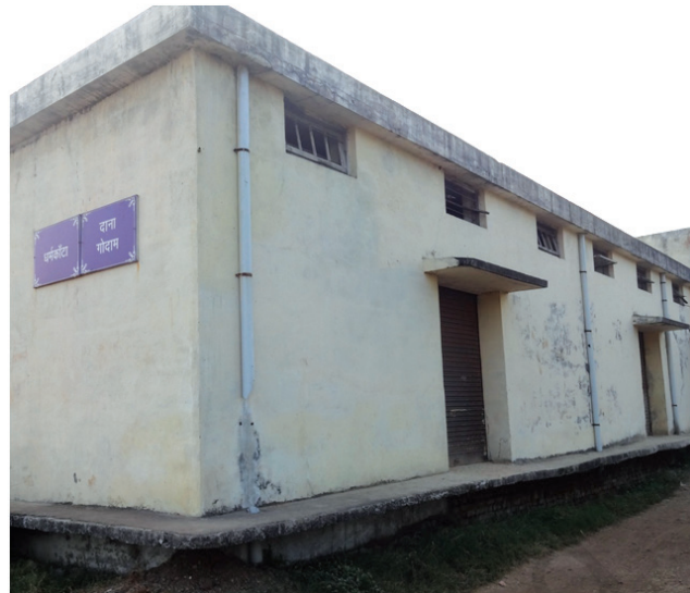
Fig. 4.15: Feed godown on raised platform
